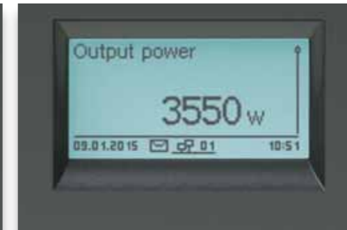
The inverter display shows the system's current performance and operating parameters.
